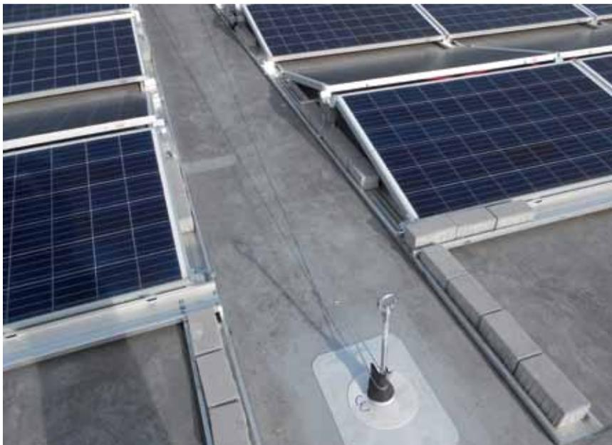
*Such connections can protect against the caterpillar effect. However, the question is how they should be dimensioned. The product in the picture can withstand up to six kilonewtons, but it undergoes deformation at 0.5 kilonewtons.*
